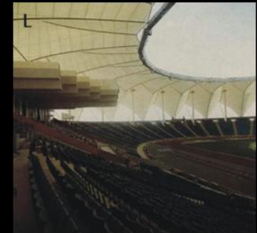
VISTA FINAL INTERIOR
