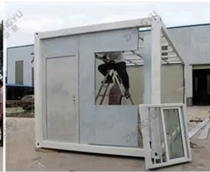
6 Install door and window
