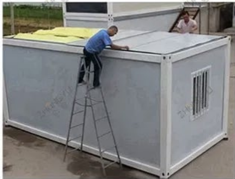
7 Laying top glass wool
