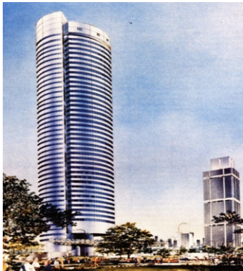
Fig 4 - Singapur Treasury Building
