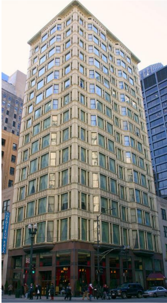
Reliance Building Chicago, 1895
