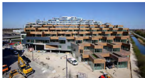
Mountain Dwellings / Big Architects / Dinamarca
